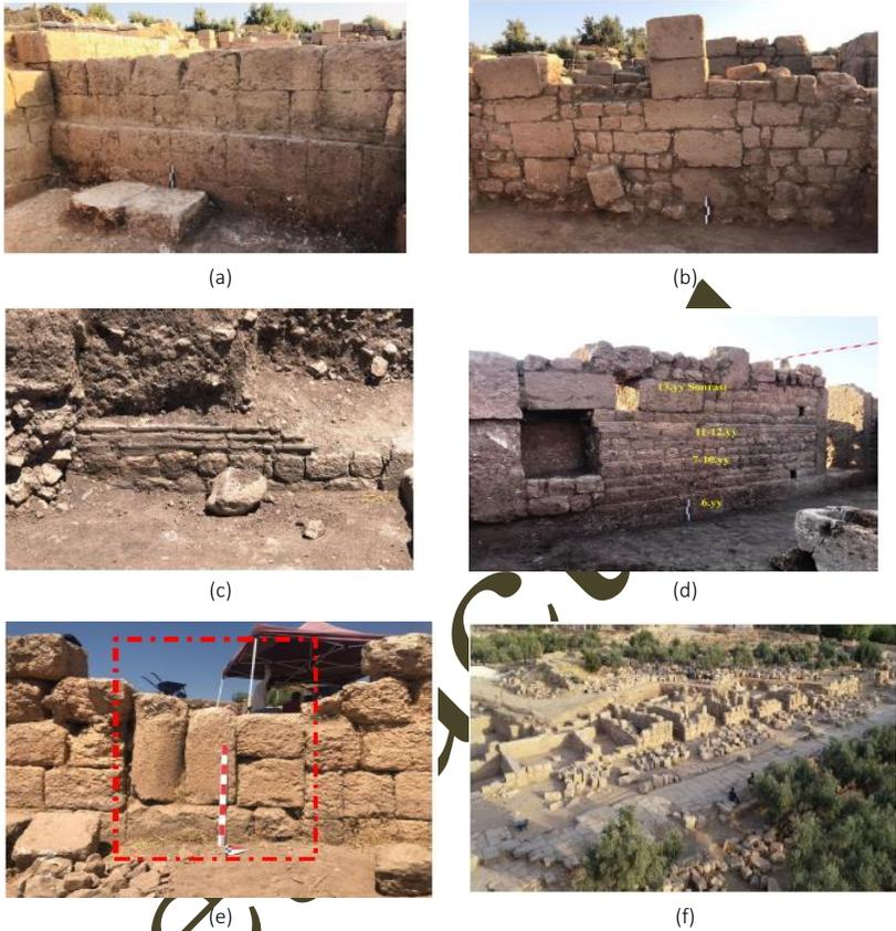
**Figure 12.** (a) Walls of the Agora Shops from the Initial Construction Phase. (b) Walls of Agora Shops from the Secondary Usage Phase - Combination of Block and Polygonal Stones. (c) Wall Utilizing Both Polygonal Stones and Bricks. (d) Chronological Sequence of Wall Techniques Used in the Shops. (e) Closed State of Shop Doors Prior to Excavation. (f) Open State of Shop Doors after Excavation.
